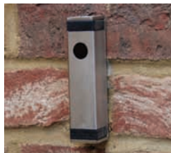
2 pairs of photocells
